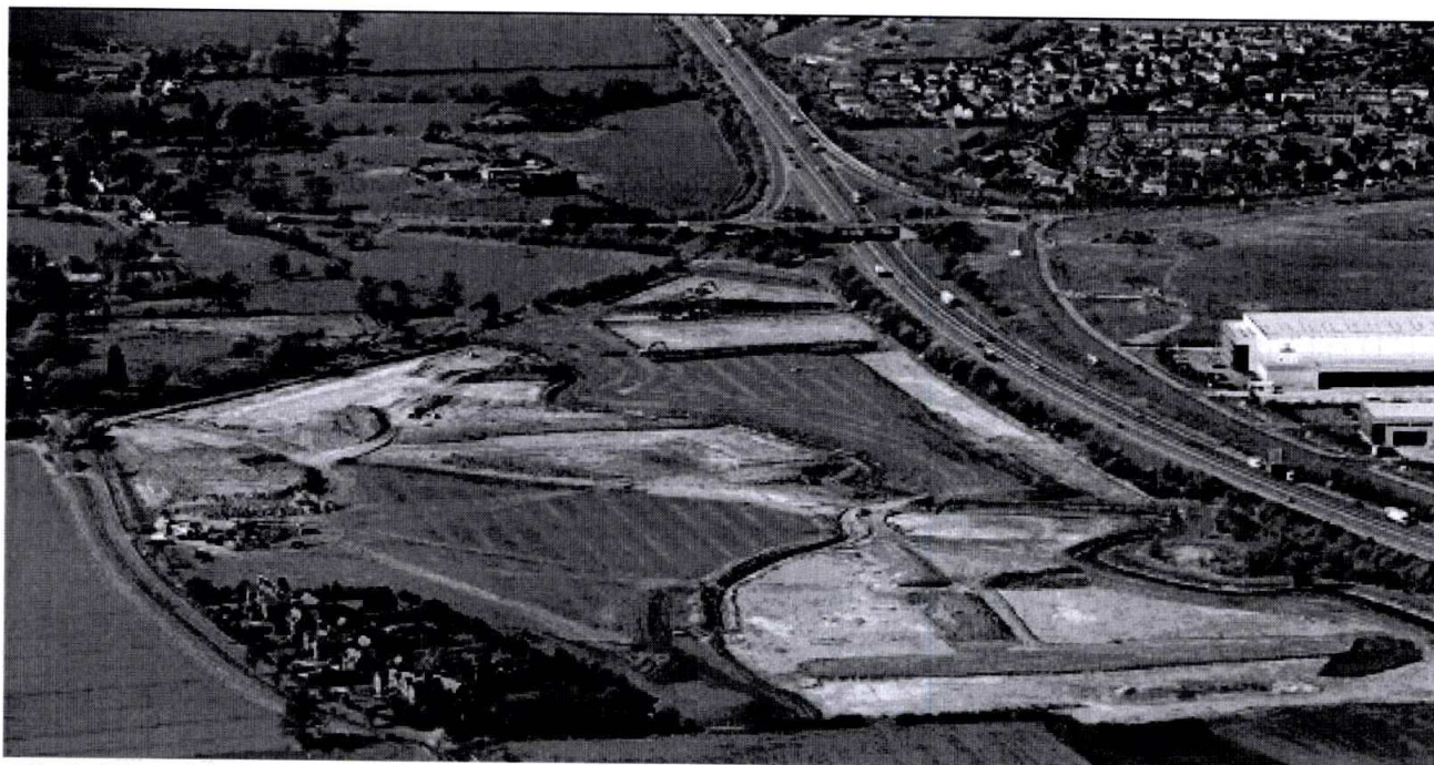
Fig 2. View of the investigation area from east during earthmoving with Harrowden (top left) and outskirts of Bedford (top right).
